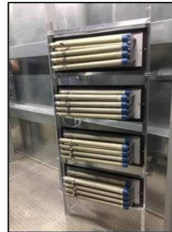
AtmosAir 508FC systems in Discharge of AHU
